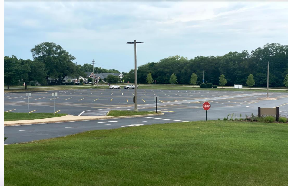
OHS North Parking Lot – After
