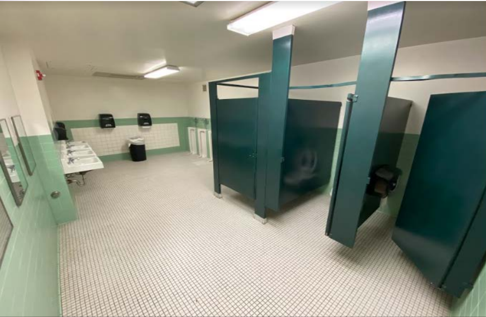
Boys Restroom Before
