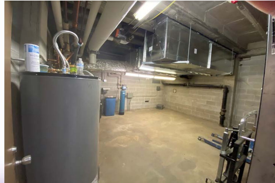
Make-up Air Unit Removed
